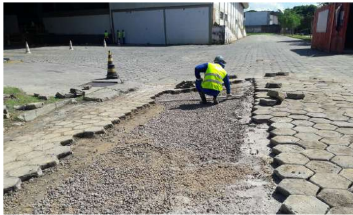
Concrete counterweight waste reuse at Manaus Plant, Brazil.
