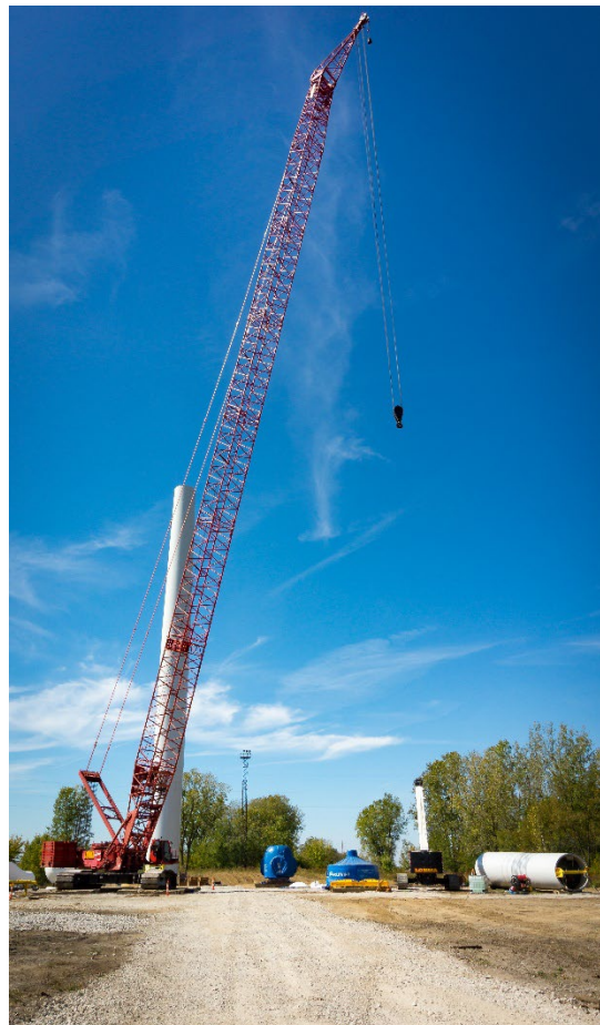
A crane mat in use
