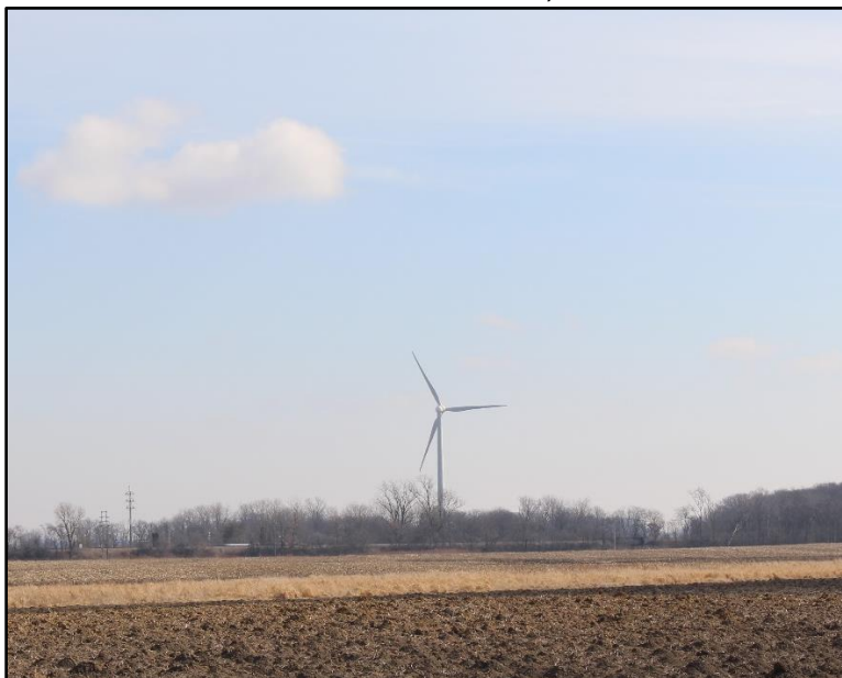
A 1.5 MW wind turbine in operation.
