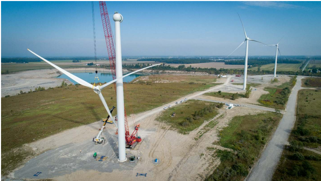
Figure 1: Crane on crane pad, flying the rotor during construction
