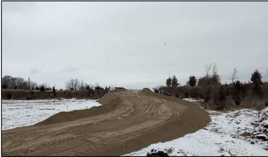
Figure 2: Dirt ramp at a wind turbine construction site
