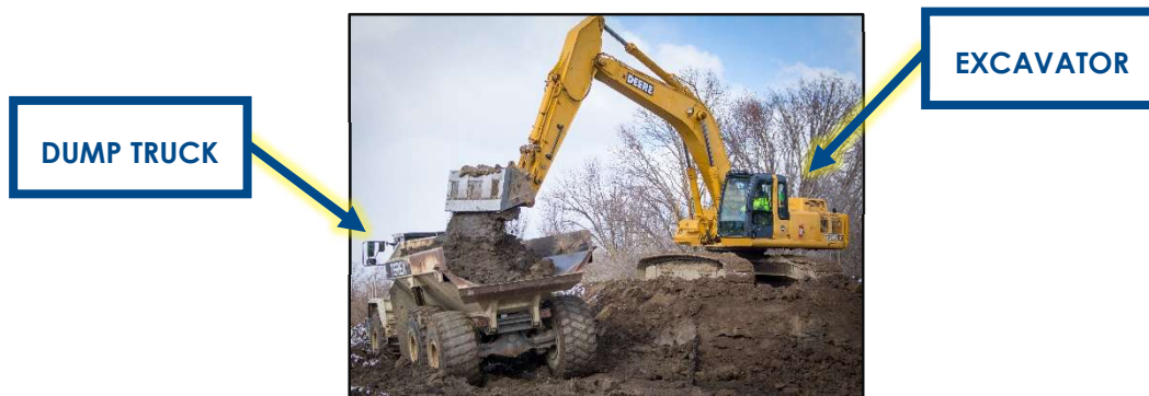
Figure 1: An Excavator loading dirt onto a dump truck.
